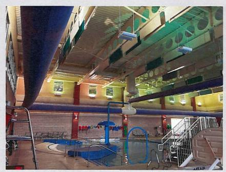
The Desert Air system, when functioning, removes air that contains chloramines and carbon dioxide from the interior of the natatorium. It then replaces with the appropriate amount of fresh air from outside of the facility. Through this process the system also dehumidifies and cools the air within the facility. Controlling this process allows for a more comfortable working environment for staff and more enjoyable atmosphere for all our facility users.
